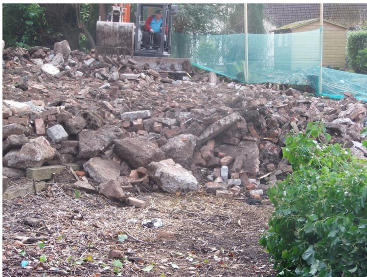
Raising of ground level
